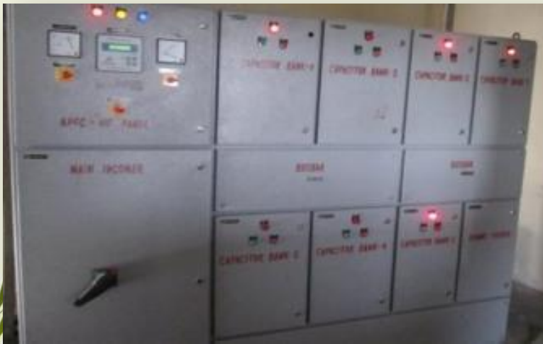
APFC panel to maintain unity power factor
