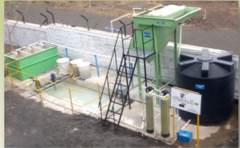
Effluent Treatment Plant
