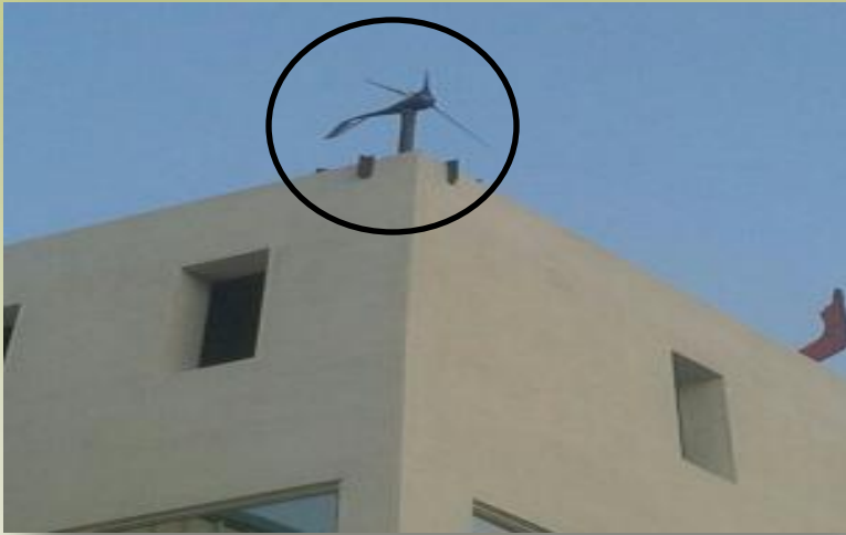
Wind Turbine for office & utility lighting
