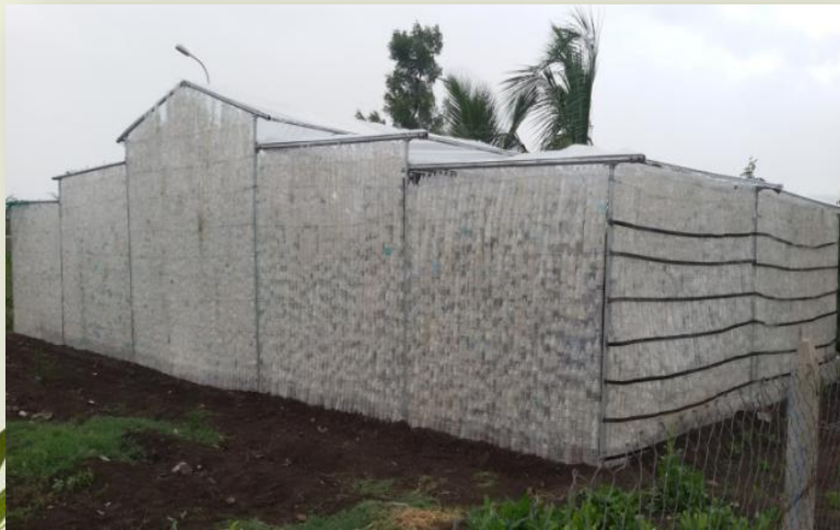
Green house constructed from recyclable & waste material
